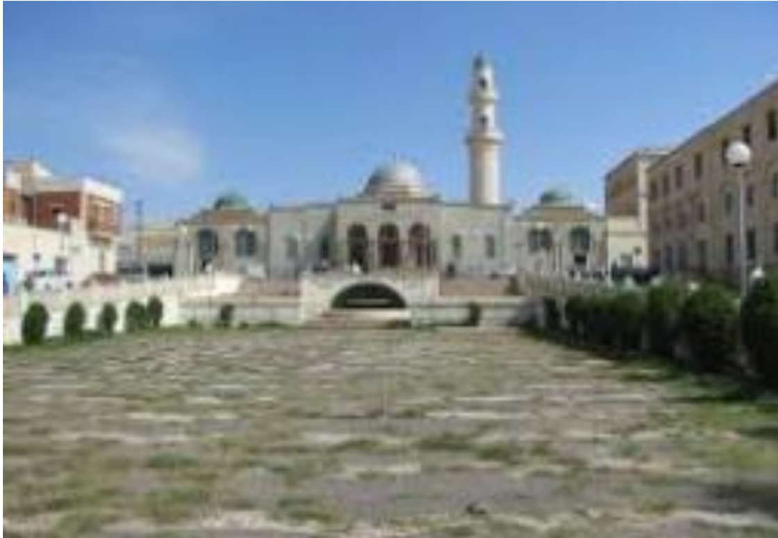
A mosque in down town Asmara
