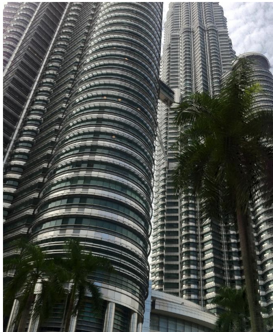
Kuala Lumpur twin towers
